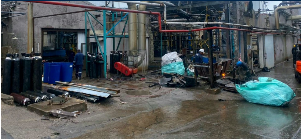
DEMOLISHING THE CURRENT FISHMEAL PLANT
