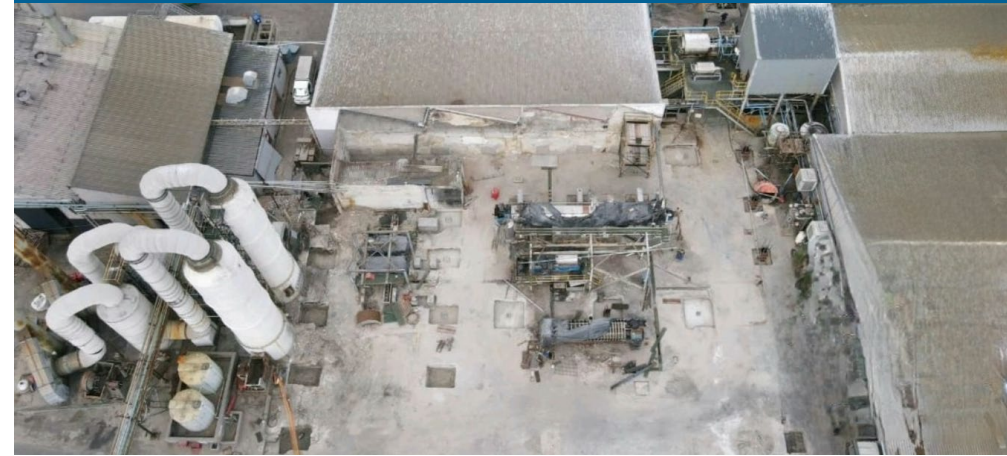
FISHMEAL PLANT UPGRADE
